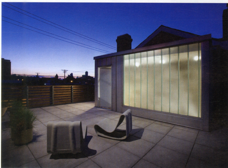
TOP Cinder block walls extend from the house to form the garden walls. The back of the fireplace, nested in the window wall, juts out into the garden and is clad in weathering steel. The rear facade is skinned in asphalt shingles.
